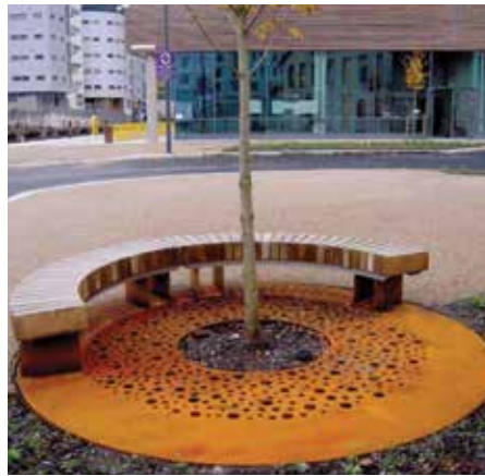
Corten tree grille and timber bench
