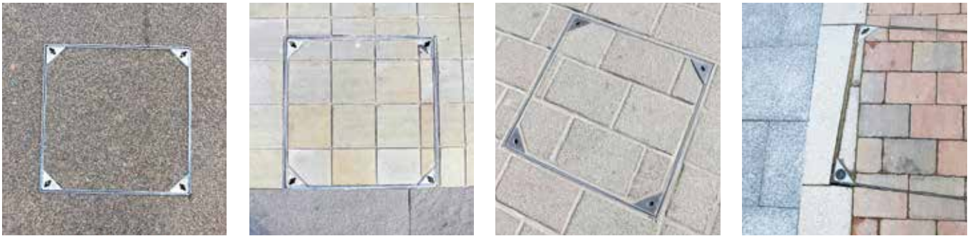
A range of well finished drain covers
